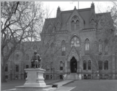
University of Pennsylvania Historic Stone Facade Repairs
